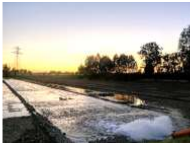
Surface irrigation system
