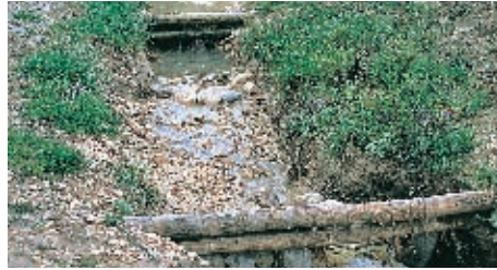
Figure 30. Small gully with spontaneous vegetation and small structures to slow down runoff velocity.
