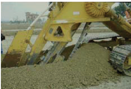
Figure 23. Digging and laying drainage pipes.
