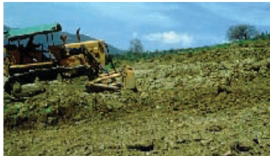
Figure 20. Levelling the site.
