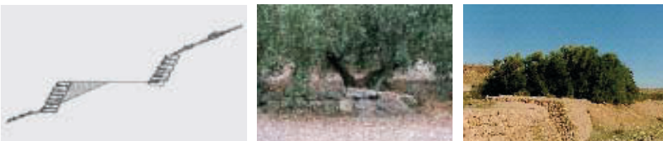
Figure 27. (A) Design of a bench terrace faced with thick stones, (B) olive orchard protected by this system and (C) traditional Jessor dyke constructed in Tunisia to harvest water and sediment (Photo: Taïeb Jardak).
